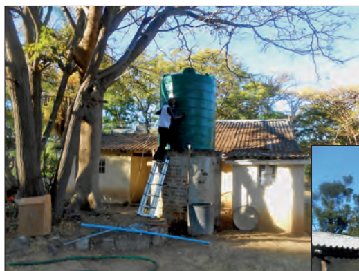
5000L water tank with solar pump installation
