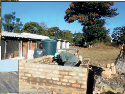
Stand for the 2000L tank being built
